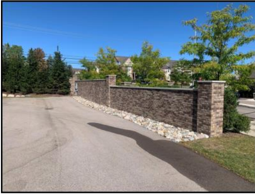
Figure E11: Huntley Manor Apartments in Novi has screening that separates Grand River, a major arterial, from residential units. Both decorative walls and landscaping in the form of trees were used to screen the homes from the street.
