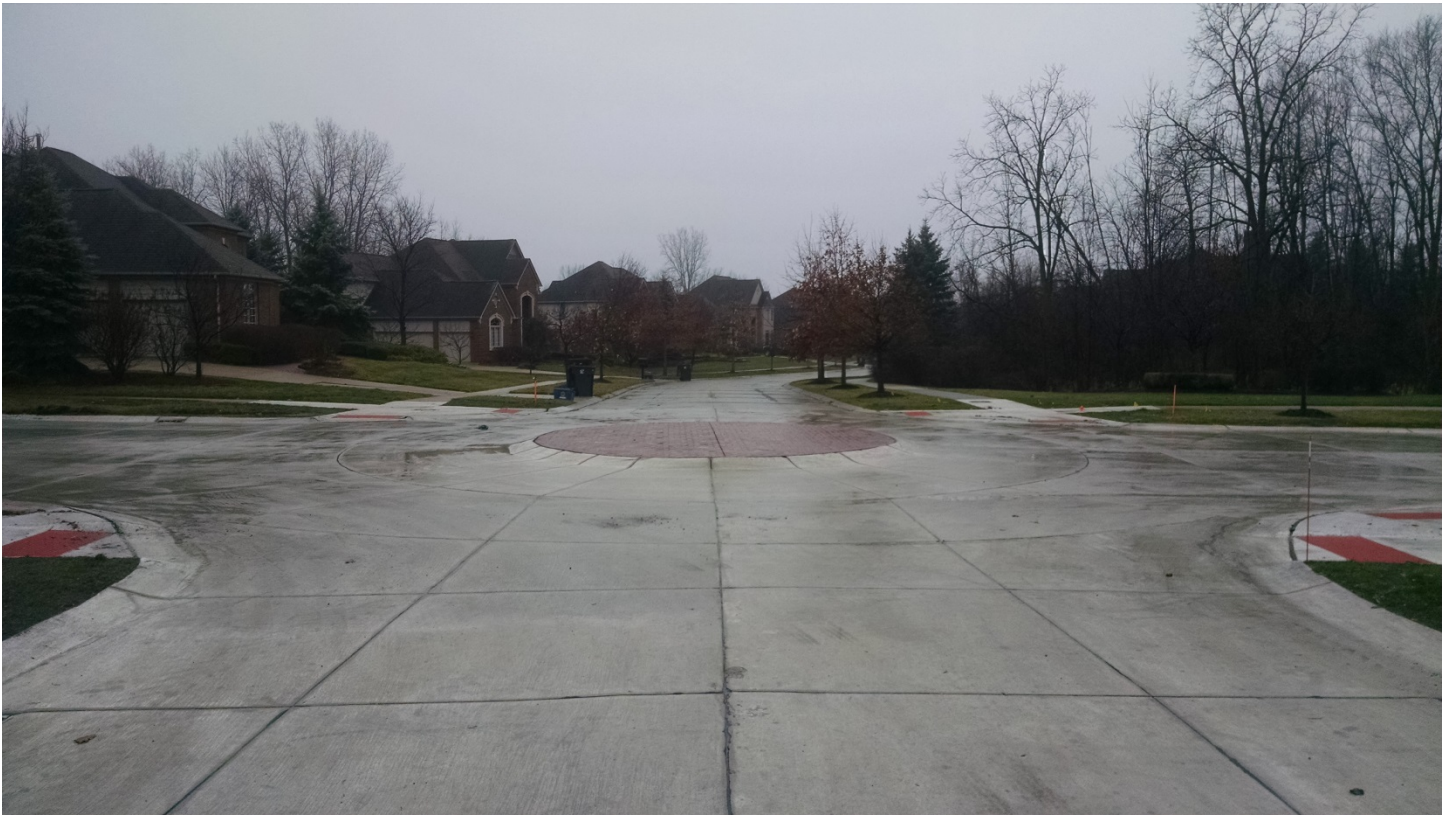
White Pines Drive at Arden Glen Court – Traffic Circle Looking East
