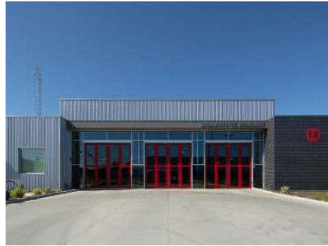
SACRAMENTO, CA FIRE STATION NO. 14
