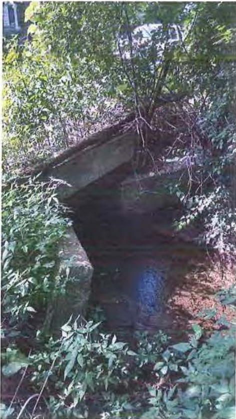
East End of Bridge
