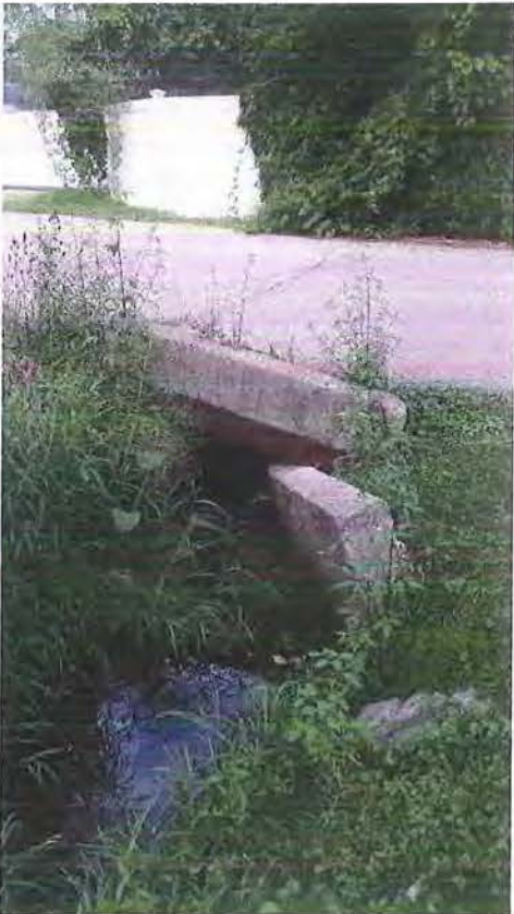
West End of Bridge
