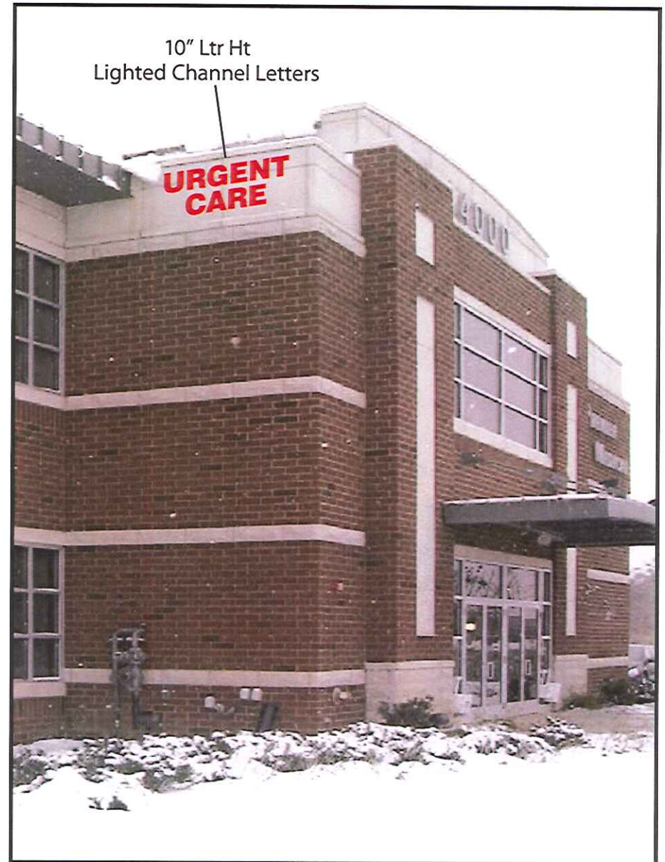
Two sets of white aluminum channel letters 10" high x 4" deep with red LED illumination (UL) and red acrylic faces, mounted on white aluminum raceways.
