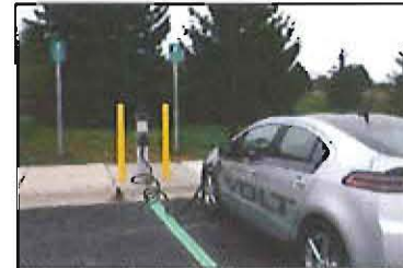
City of Novi electric vehicle charging station located at 45125 W. Ten Mile Road, Novi Police Headquarters. Chevy Volt courtesy of Marty Feldman Chevrolet.
