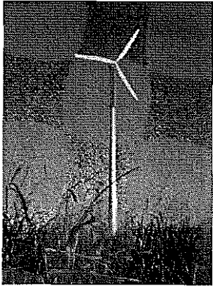
Entegrity Wind Systems 50kW turbine
