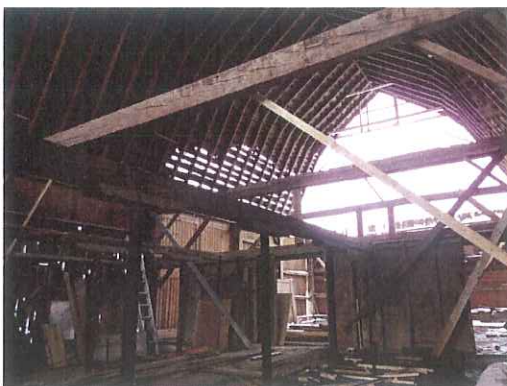
West Barn Interior View
