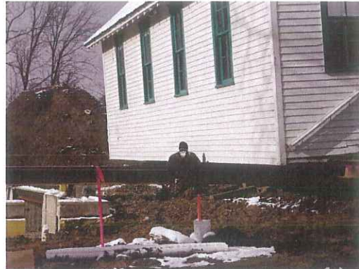
Township Hall Was Moved Using Steel Beams
