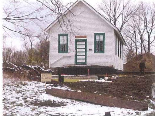
Township Hall Prior to Being Placed on its New Foundation
