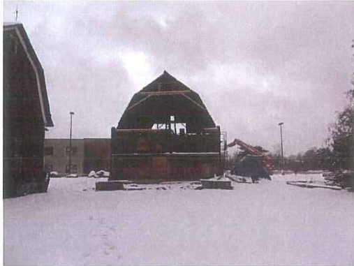
West Barn Exterior View
