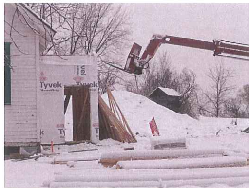
Restroom Addition Under Construction
