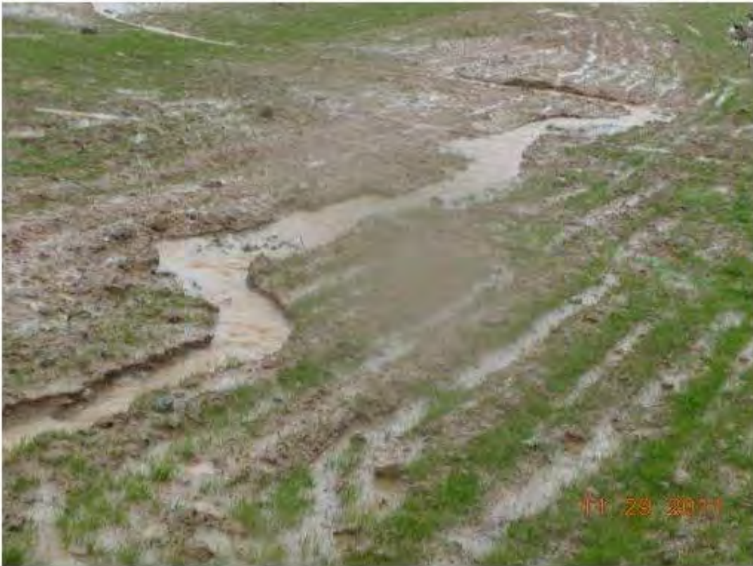
Gullies are forming on the sloped area. Silt fence has been undermined in a few places.
