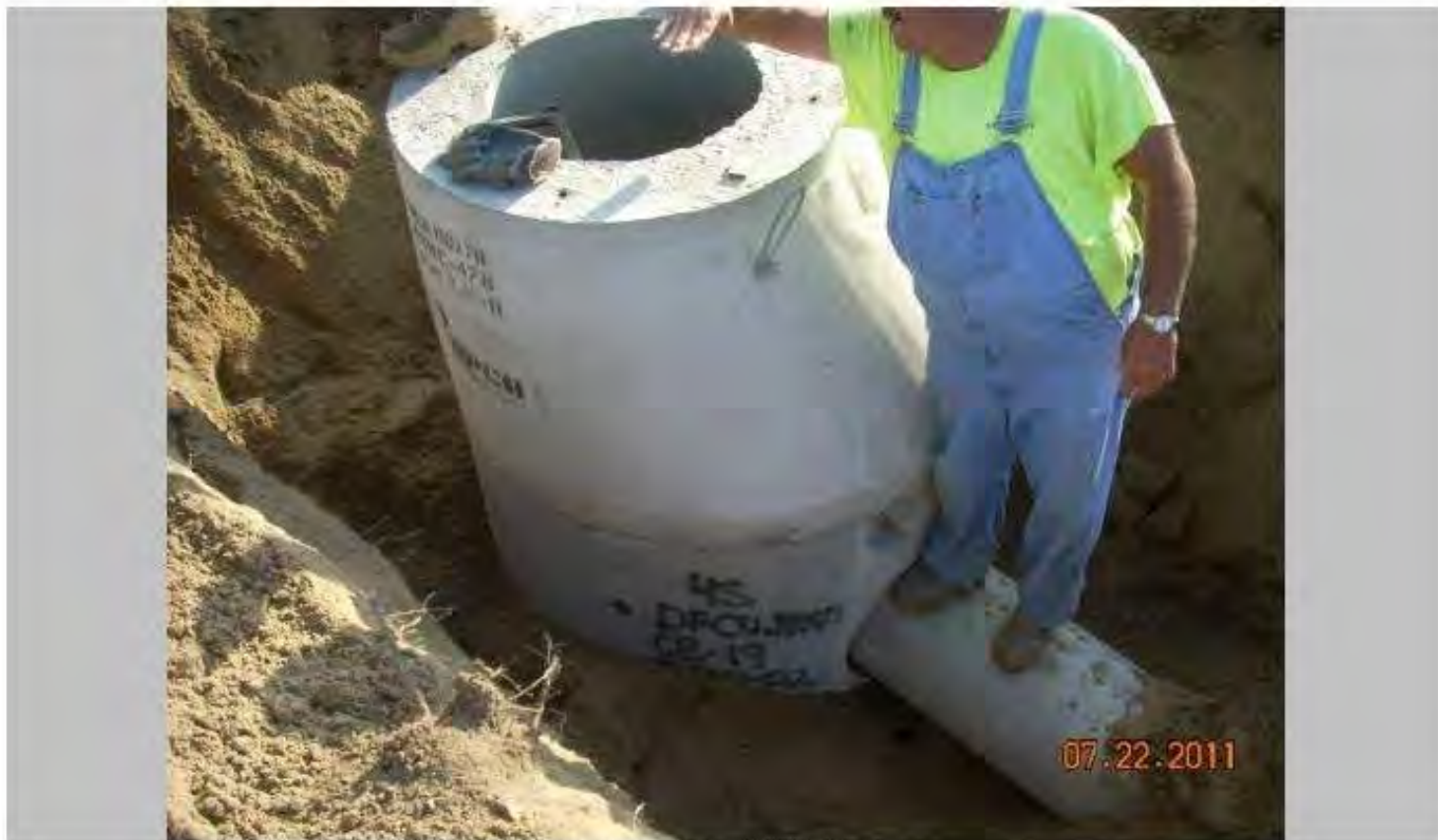
CATCH BASIN #19 ASSEMBLED
