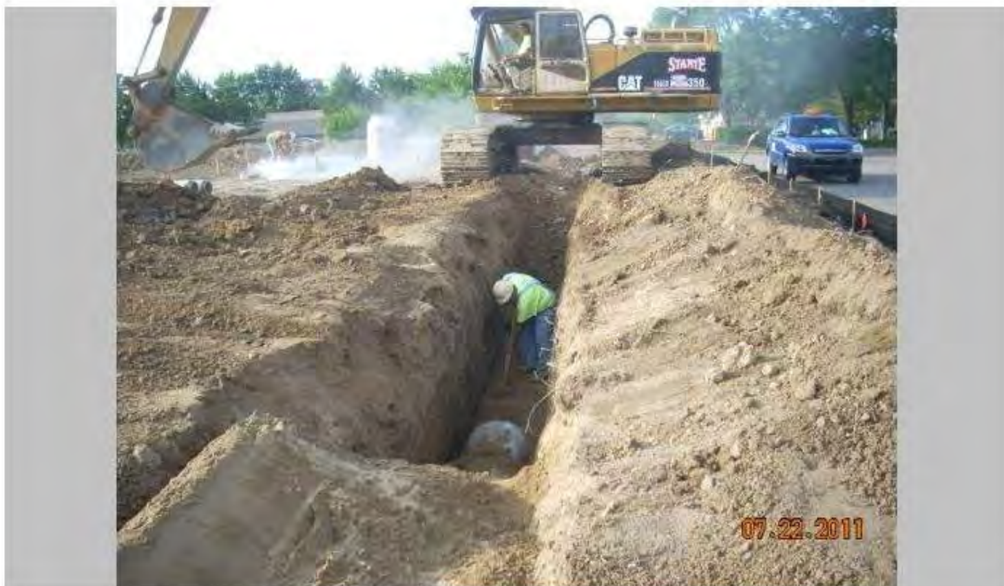
LAYING 12" RCP FROM CATCH BASIN #19 TOWARD CATCH BASIN #18
