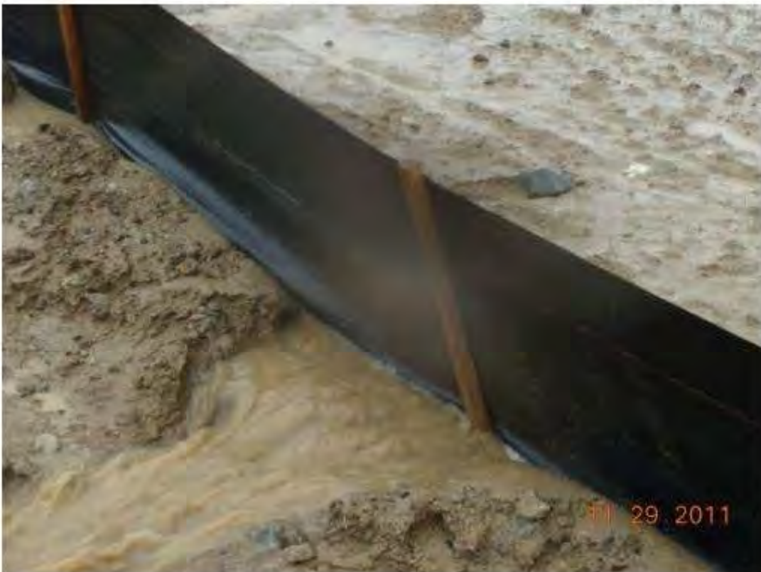
Gullies are forming on the sloped area. Silt fence has been undermined in a few places.
