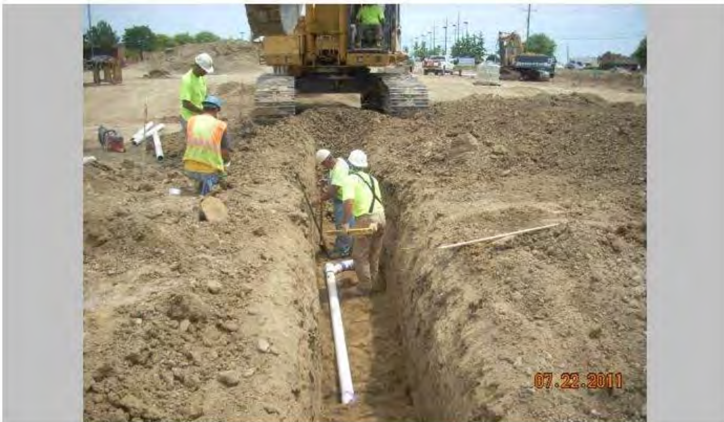
LAYING ROOF CONDUCTOR LEADS FOR THE CANOPY
