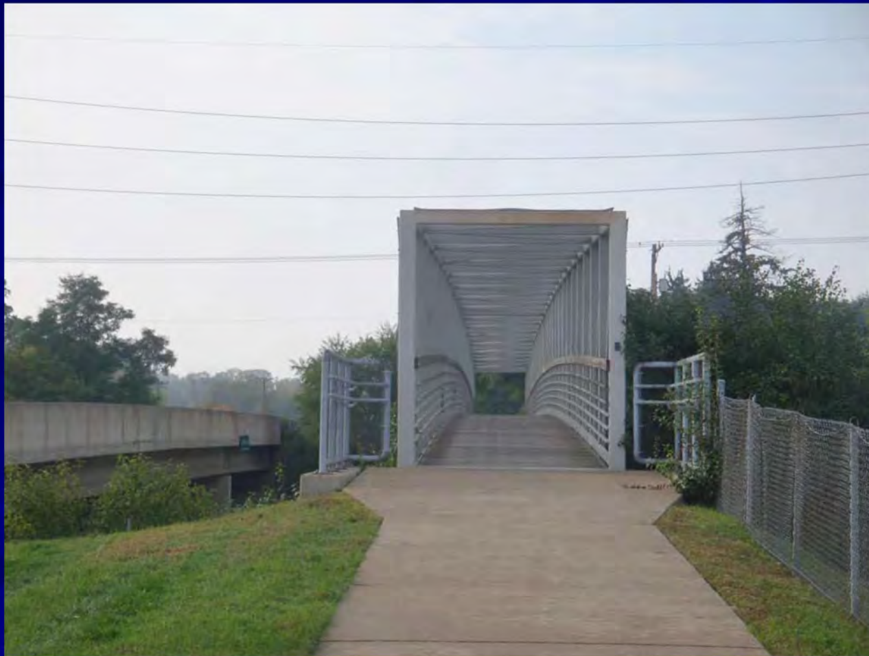
Bridge - 8 foot wide
