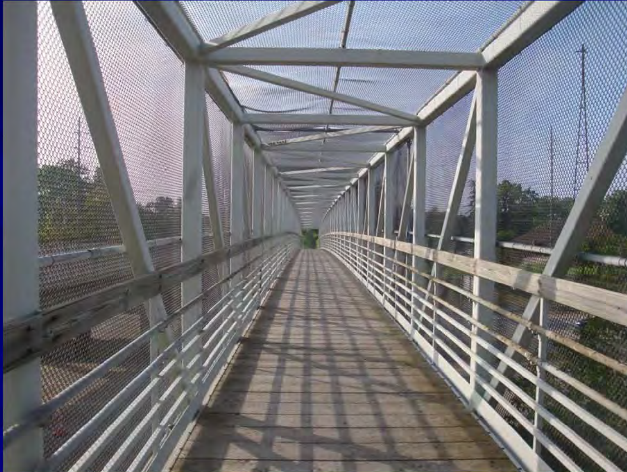
Enclosed bridge, wood deck
