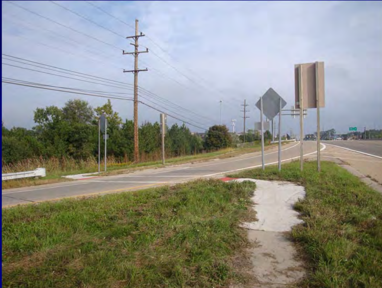
Sidewalk crossing of free flow ramp
