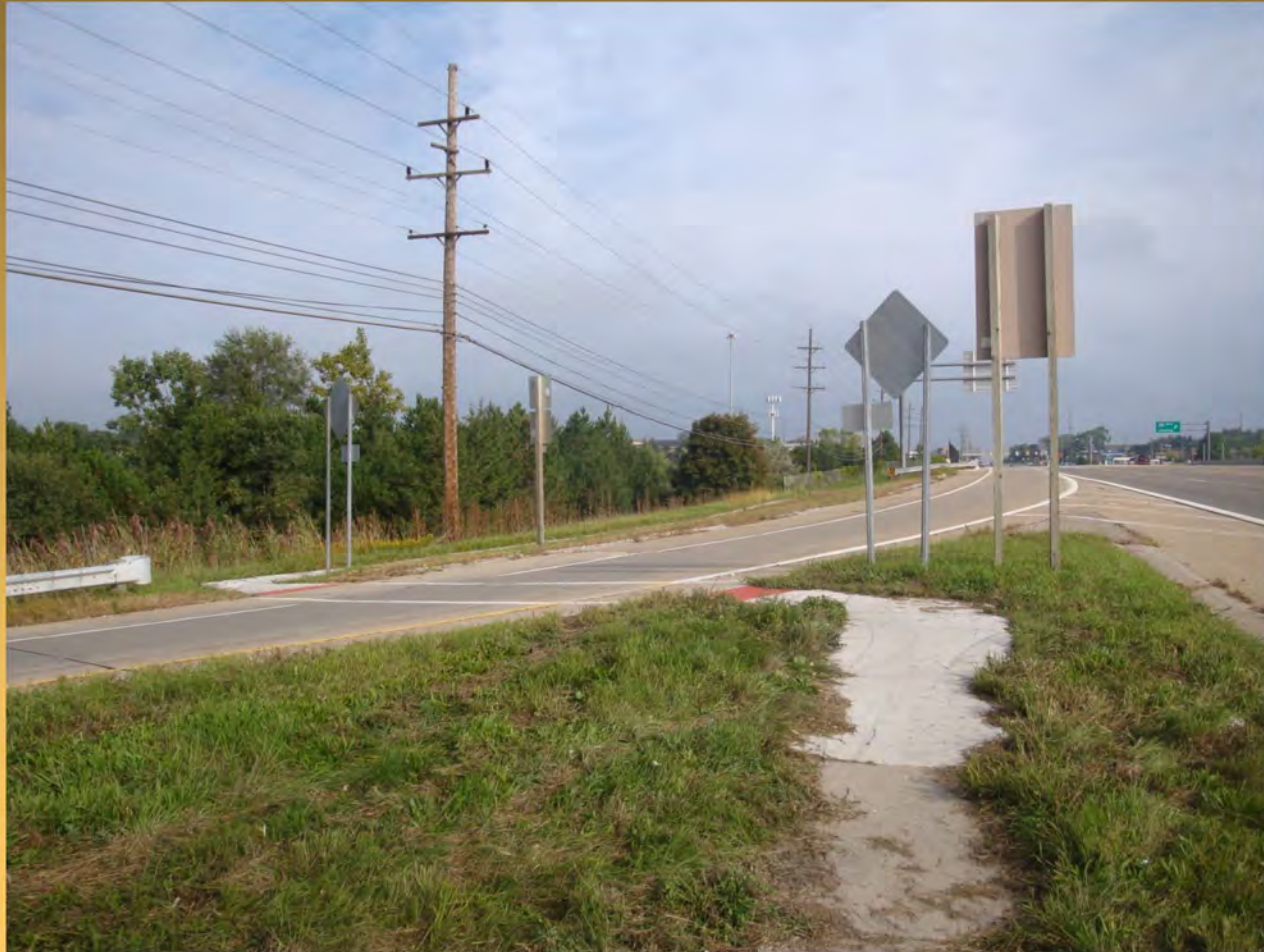
Sidewalk crossing of free flow ramp
