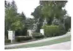
Masonry Piers and Walls
