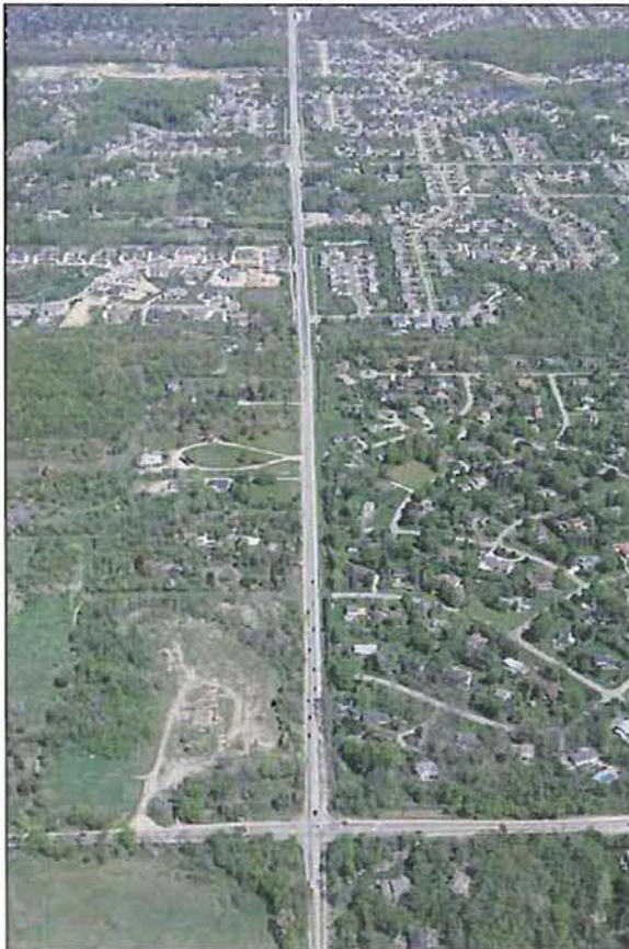
Figure 21 Beck Rd. looking north from Eight Mile Rd.
