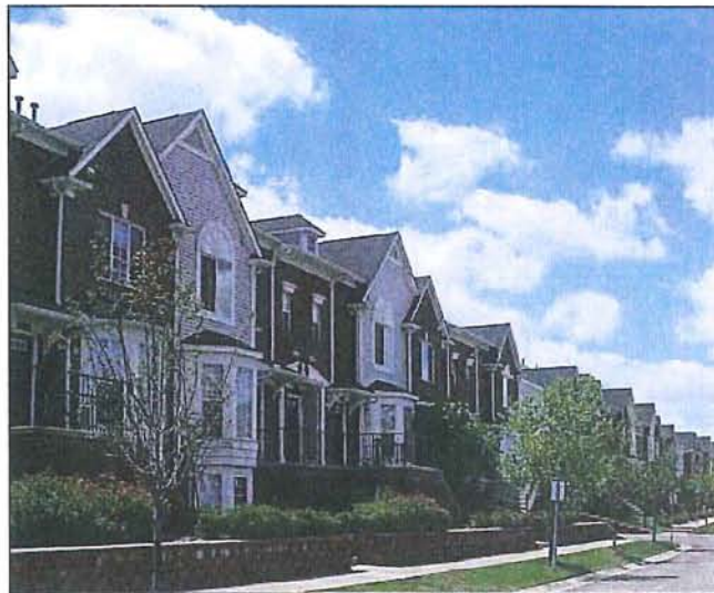
Figure 24 - Example of multiple-family residential at 4 dwelling units per acre ( Brownstone Apartments 2009 ).
