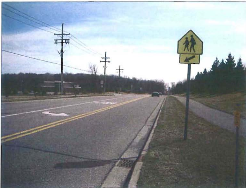
Figure 8. Southbound School Crosswalk Warning Sign Past Crosswalk
