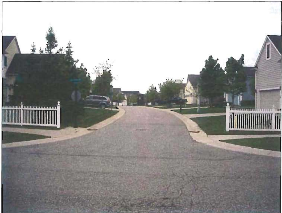
Figure 5. View to East Down Muir Lane
