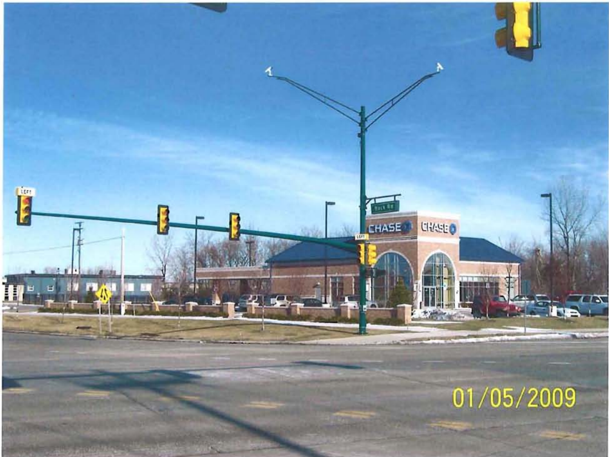
View of NE corner where two additional decorative poles would be installed.
