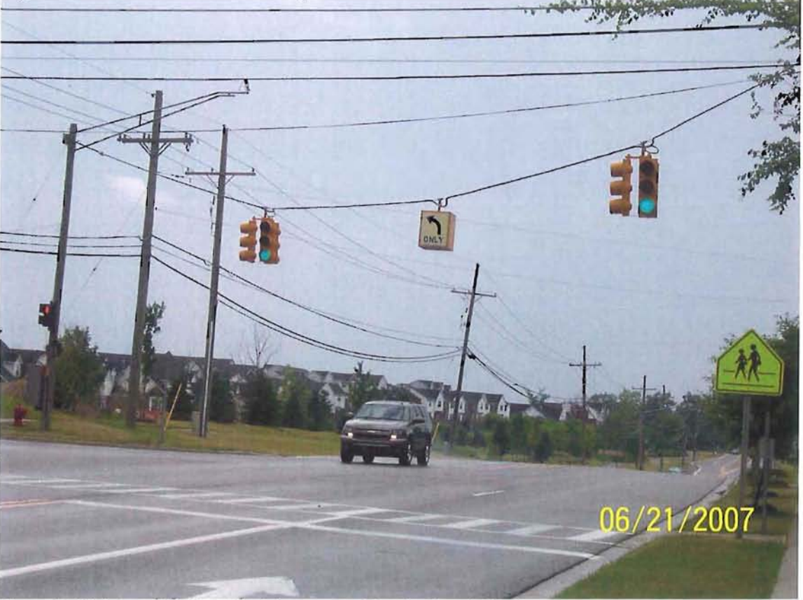
Figure 2. Thirteen Mile Road looking west at Meadowbrook Road
