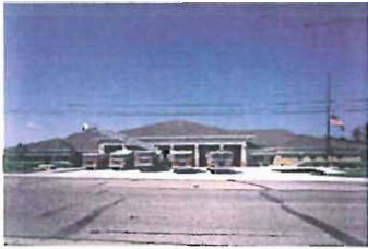
CENTRAL FIRE STATION (2003) Delta Township
