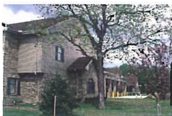
PUBLIC SAFETY BUILDING (2002) Northfield Township
