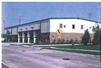
INTERIM FIRE STATION/DPW (2002) City of Wayne
