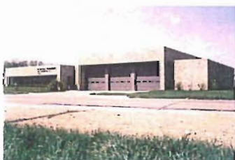
HEADQUARTERS FIRE STATION (1987) Clinton Township
