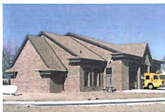
FIRE STATION NO. 3 (2005) Brandon Township
