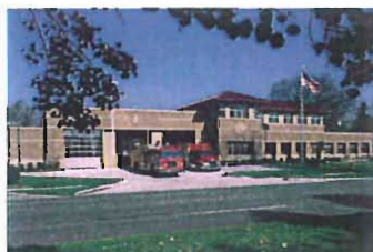
FIRE STATION NO. 3 (2005) City of Farmington Hills
